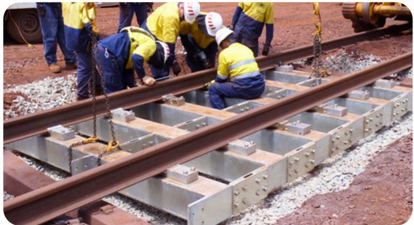
Installation of INFINITY 'LS' weighing system in curved track
